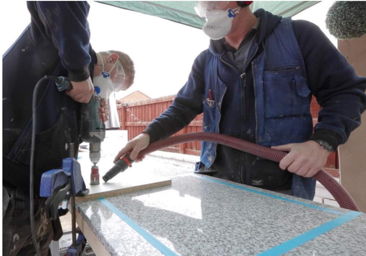
Builders cutting Howdens granite on site
